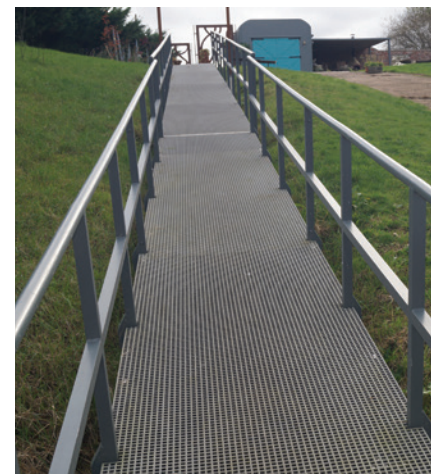
The mains drains are located at the top of the walkway; an incline of 7.5m. The walkway also moves up and down with the rise and fall of the water
