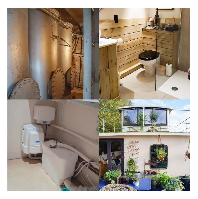
This clever installation takes the toilet and basin waste out one way to the sewage tank on board and the water from the other appliances in another direction to be pumped out of the boat in to the Thames. A further en-suite in the master cabin is powered by a Saniplus for a bath, toilet and basin.
